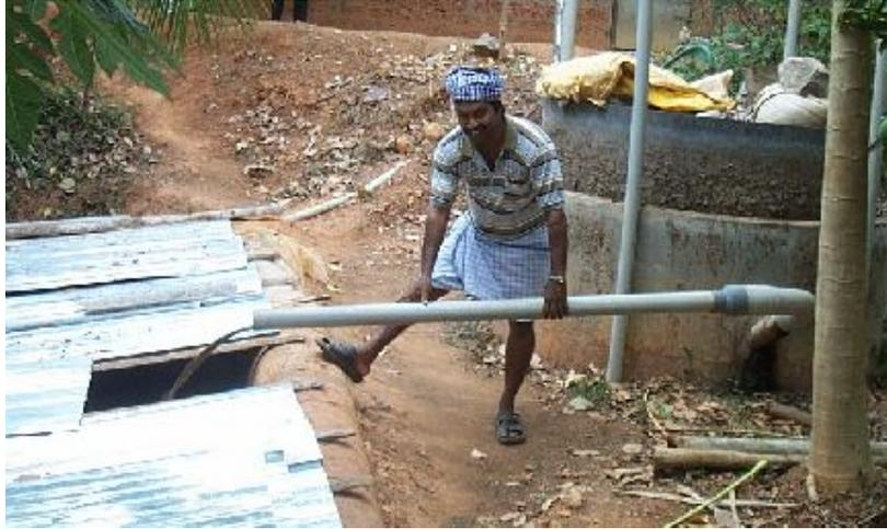
**Figure 2 : Spent slurry being collected in a tank for distribution**
